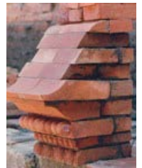
Over 23,000 bricks were used in rebuilding the Mandap
