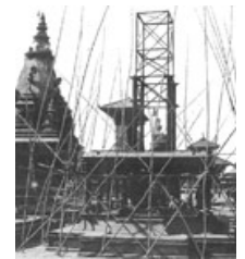
Steel structure completed in 1987
