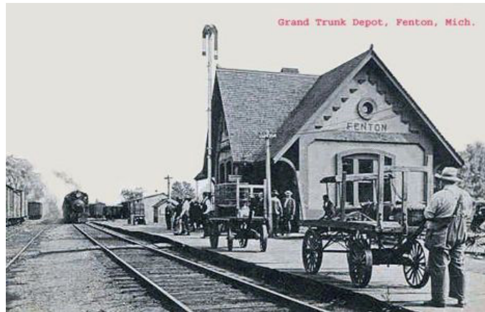
Grand Trunk Railway depot
